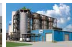
REG Okeechobee Okeechobee, FL Research Facility
